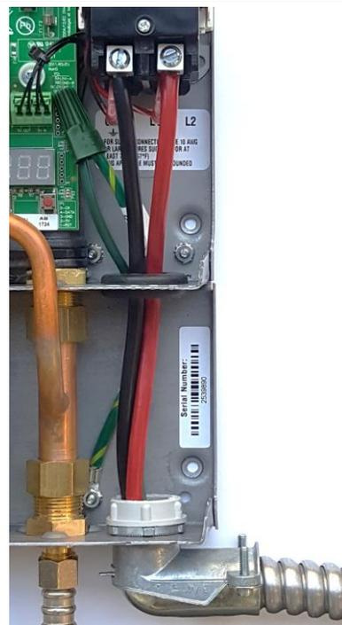
**2.** The power leads are to be secured to the L1 and L2 or L and N connectors on the terminal block or relay. The ground lead is to be secured to the GND connector on the block or the green ground wire with the provided wire nut.
