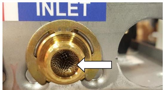
**3.** Remove the cover. Connect the pre-assembled inlet and outlet pipes to the heater (**do not overtighten compression fittings**) and fully open the inlet and outlet ball valves. Check the system for water leaks at all plumbing connections. If a leak is present at the compression fitting, **slowly** tighten compression nut until it stops – **do not overtighten**.
