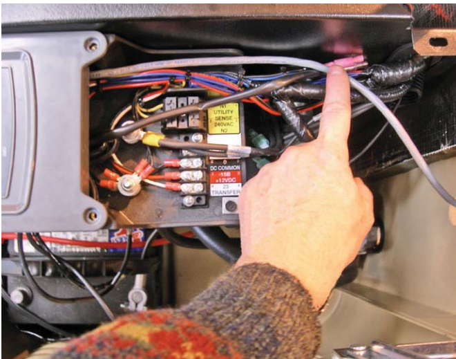
Figure 6B — Route Wire
