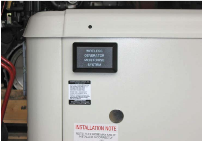
Figure 3 — Mount Transceiver
