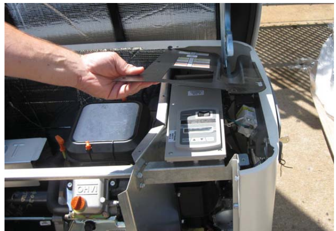
Figure 1 — Remove Control Panel Cover
