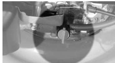
Fuel shutoff valve closed.
