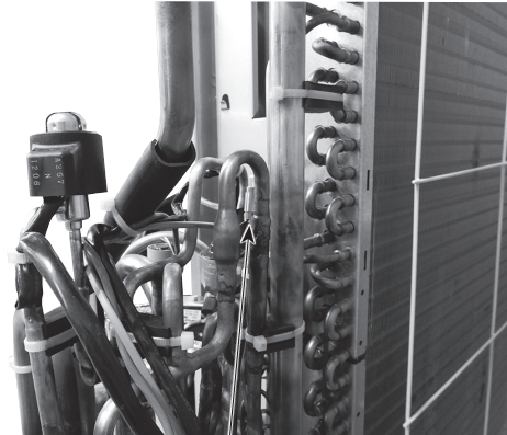
Thermistor <Outdoor liquid pipe> (TH3)
