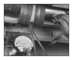
3 The airflow is regulated by a balancing damper located inside the collar of the AEV. Adjust the "Supply Air Out" damper until you reach the desired velocity. Follow the previous steps to adjust the "Exhaust Air Out" damper.
