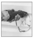
1 Using the collar of the outside hood, outline the intake & exhaust holes to be cut. The holes should be slightly larger than the collar to allow for the thickness of the insulated flexible duct. Cut a hole for both the intake and exhaust hoods.
