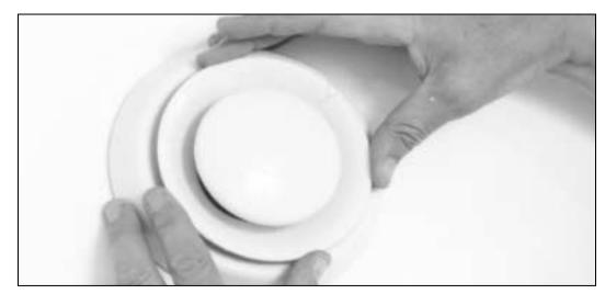
4 Push the Fantech grille {MGE (metal) or PGE (plastic)} into the optional mounting collar or directly into installed elbow.
