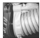
2 Working from a closet, attic or inside your joist wall, run the length of ducting required for the proper grille location and cut a hole in the gyprock. Fasten the mounting collar (optional) to the ducting and fasten the collar to the wall or ceiling with screws.
