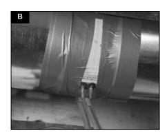
1 For this flow measuring station, cut the duct and place the flow measuring station between each station. Make sure that the flow measuring station's air direction arrow points in the direction of the airflow. Secure the flow measuring station with duct tape.
