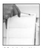
3 Push the hood into the opening. Attach the hood to the outside wall with mounting screws. Repeat the installation procedure for both the Supply and Exhaust hood.
