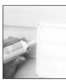
4 Using a caulking gun, seal around both hoods to prevent any leaks.
