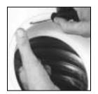
**3** The Fantech grille {MGE (metal) or PGE (plastic)} airflow can be adjusted by rotating the inside unit. It is recommended that the grilles be completely opened at first and then adjusted later as needed.
