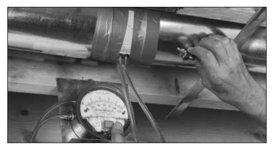
• The balancing procedure consists of measuring the exhaust air leaving the system and the supply air entering the system and ensuring that these two are equal. A deviation of 10% or less is acceptable. In such cases, it is recommended to have a greater amount of exhaust air than supply air as so to increase the supply air's temperature.
