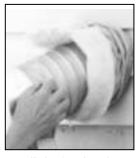
2 Pull the insulated flexible duct through the opening until it is well extended and straight. Slide the duct's inner vinyl sleeve over the hood collar and secure, pull the insulation over the duct and then the vapour barrier over the sleeve and secure with duct tape.
