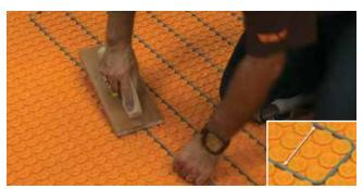
Embed the heating cables between studs, at spacing of 3 studs.
