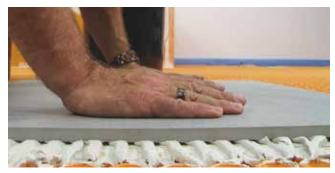
Using Schluter SET™, ALL-SET™, FAST-SET™, or unmodified thin-set mortar, tile can be installed over DITRA-HEAT and DITRA-HEAT-DUO immediately; no need for self-levelers.
