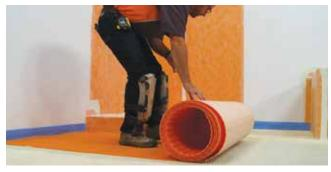
1 Apply DITRA-HEAT or DITRA-HEAT-DUO to the floor, fleece side down. Solidly embed the matting into the mortar.
